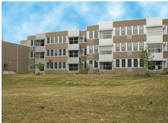
The Vegetated Infiltration Basin beneath this playfield manages rooftop runoff from the adjacent school building, Philadelphia, PA
