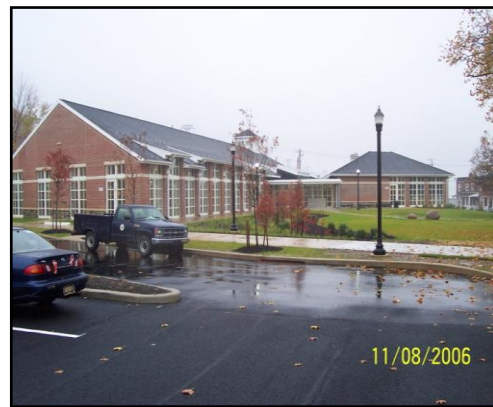
Porous asphalt parking lot in Wilm., DE
