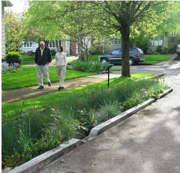
Urban application of a vegetated curb extension in Portland, Oregon (Source: www.artfulstormwater.net )
