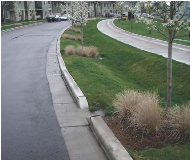
Curb opening to grass swale in residential development
