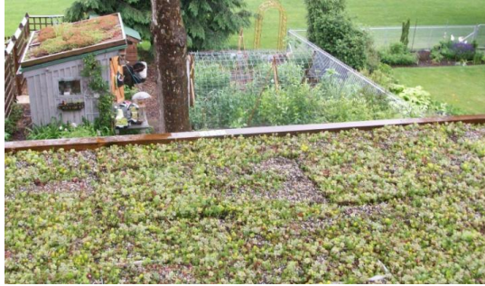
Residential vegetated roof in the City of Lancaster (Source: LiveGREEN)
