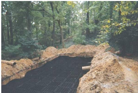
Subsurface Infiltration Bed using Rainstore™ blocks for storage media, Washington National Cathedral, DC
