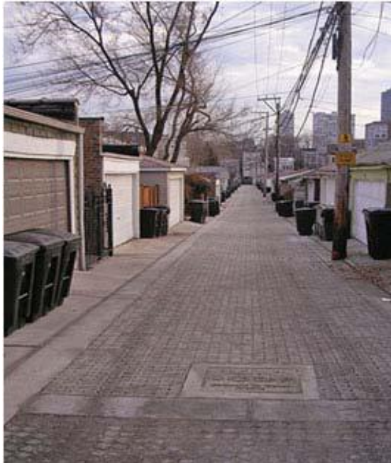
Green Alleyway in Andersonville, Chicago IL, Source: Chicago Department of Transport
