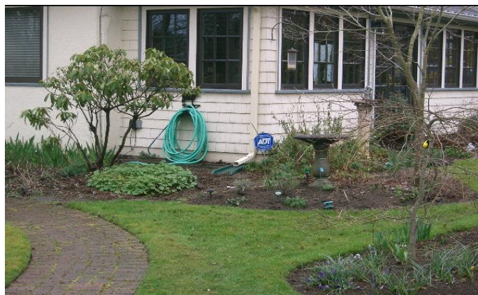
Residential downspout disconnect in Portland Oregon (Source: Portland Stormwater Website)
