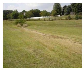
Conventional stormwater basins help control flooding during large storms, but often do little else to reduce the harmful effects of stormwater.
