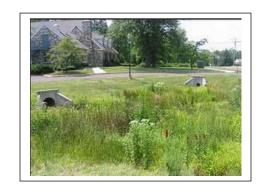
transforming a conventional basin into a natural ecosystem capable of providing habitat, improving the water quality, and providing aesthetic value. A long-term benefit is the reduction of costs required to maintain these basins.
