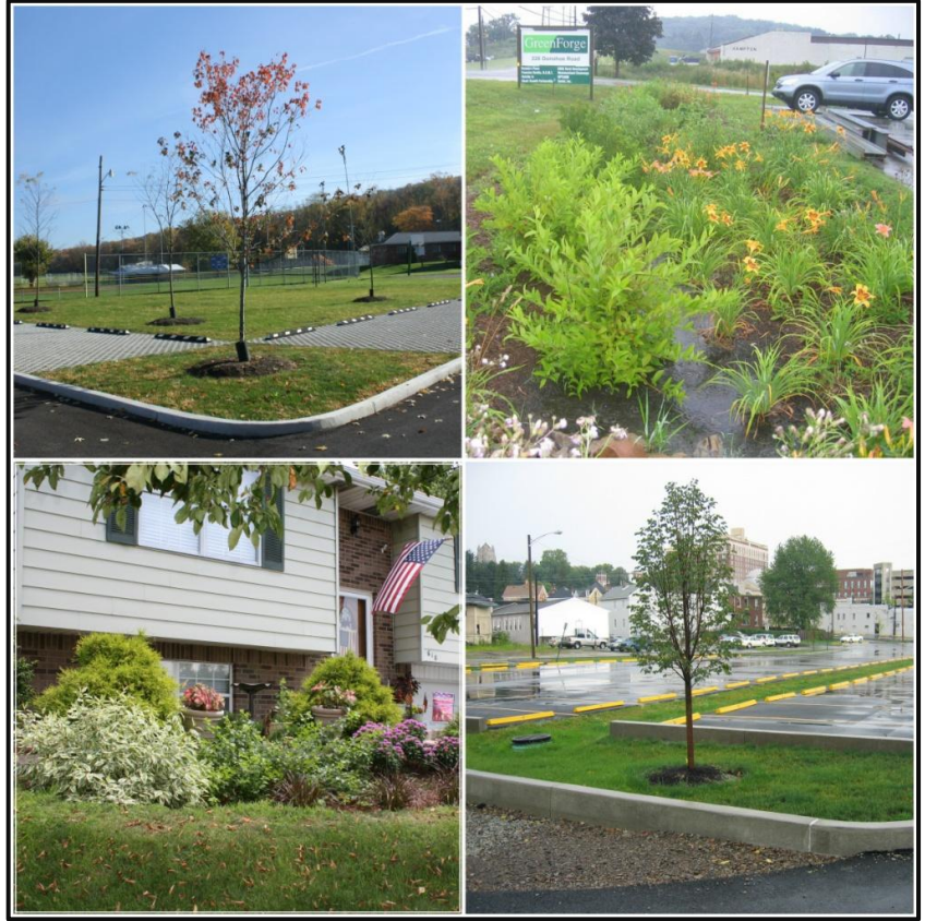
Figure 13: Local examples of Structural BMPs. Derry Borough parking with porous pavers (top left), a rain garden at Green Forge (top right), a residential rain garden (bottom left), and an adjustment to a parking lot in Greensburg. (Source: Westmoreland Conservation District)
