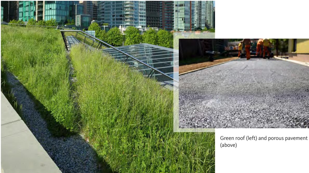
Green roof (left) and porous pavement (above)
