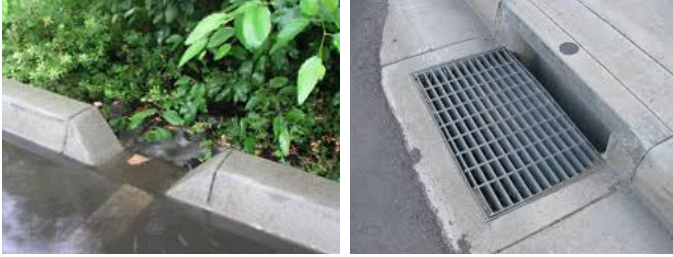
A curb cut for a bioswale vs. a common inlet
