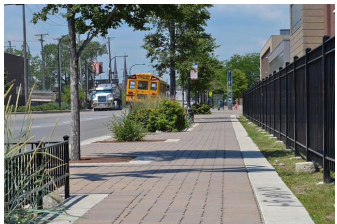
Figure D-2-1. Retrofit projects often combine multiple practices, such as bioretention and rain gardens, bioswales and pervious pavement to improve stormwater management in a developed area. Photos: Center for Neighborhood Technology, Flickr
