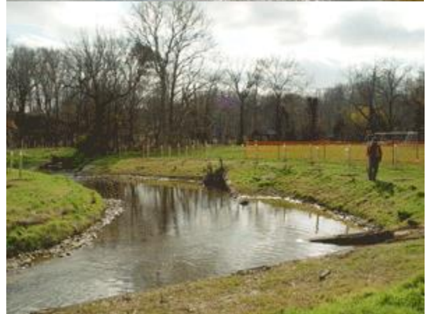
Figure A-9-1. Stream restoration projects can improve the health of aquatic resources and can be one of the more cost-effective practices to reduce nutrient and sediment loads in urban watersheds. A stream prior to restoration (top) that has an eroded stream bank and channel can be restored so that natural processes reduce the erosive energy of the stream flow during storm events. The bottom picture is the same stream shortly after completion of the project. Photos: US Fish and Wildlife Service
