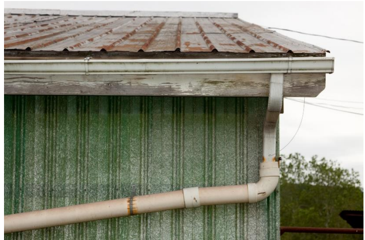
Figure A-7-1. Gutters, or roof runoff structures, can divert precipitation away from areas where animals and manure are present, which keeps the runoff water clean. Photo: USDA NRCS
