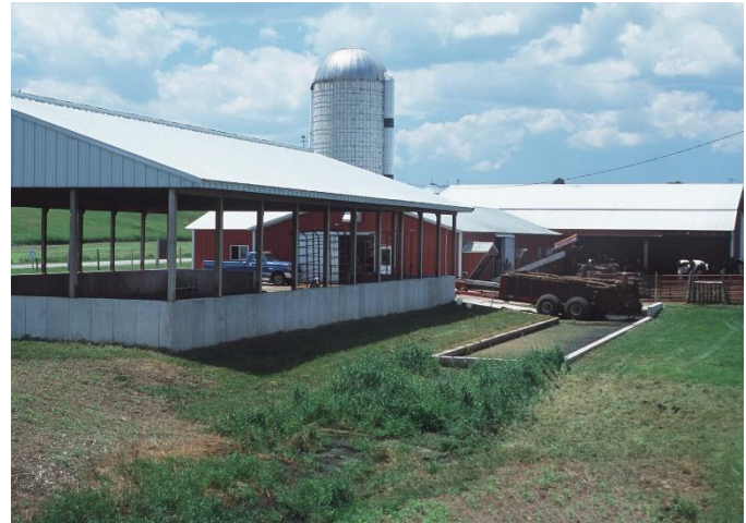
Figure A-6-1. This dry manure stacking facility (at left in photo) is used to store manure until the farmer is ready to treat, transport or apply it. The pictured facility has a roof and concrete walls to prevent manure loss or runoff. Source: NRCS Photo Gallery
